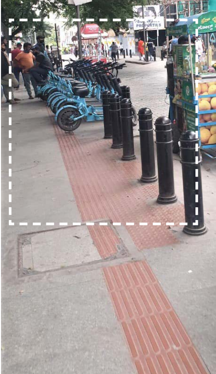
Image 2.21 Obstructions on tactile pathway
