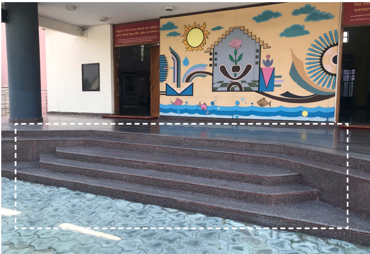
Image 2.3 Absence of adequate visual contrast in steps
