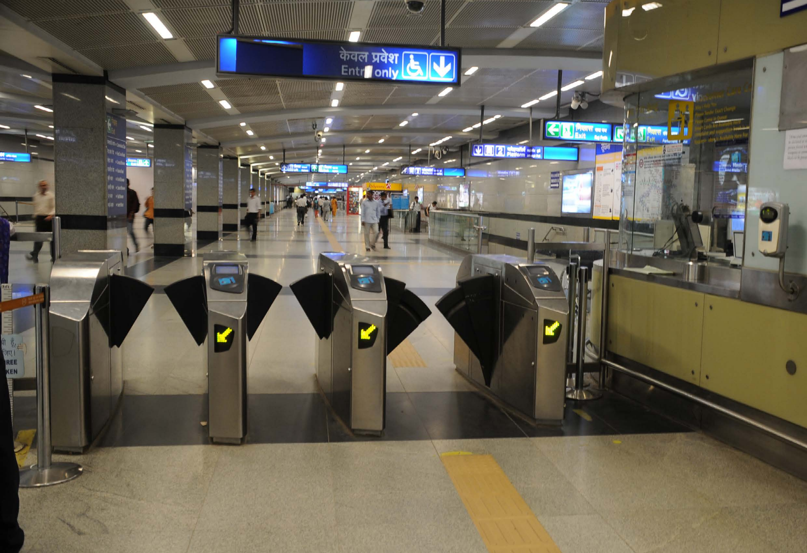
Image 6.28 Accessible automatic fare collection (AFC) system in Metro Stations Photo Credits: Dr. Gaurav Raheja
