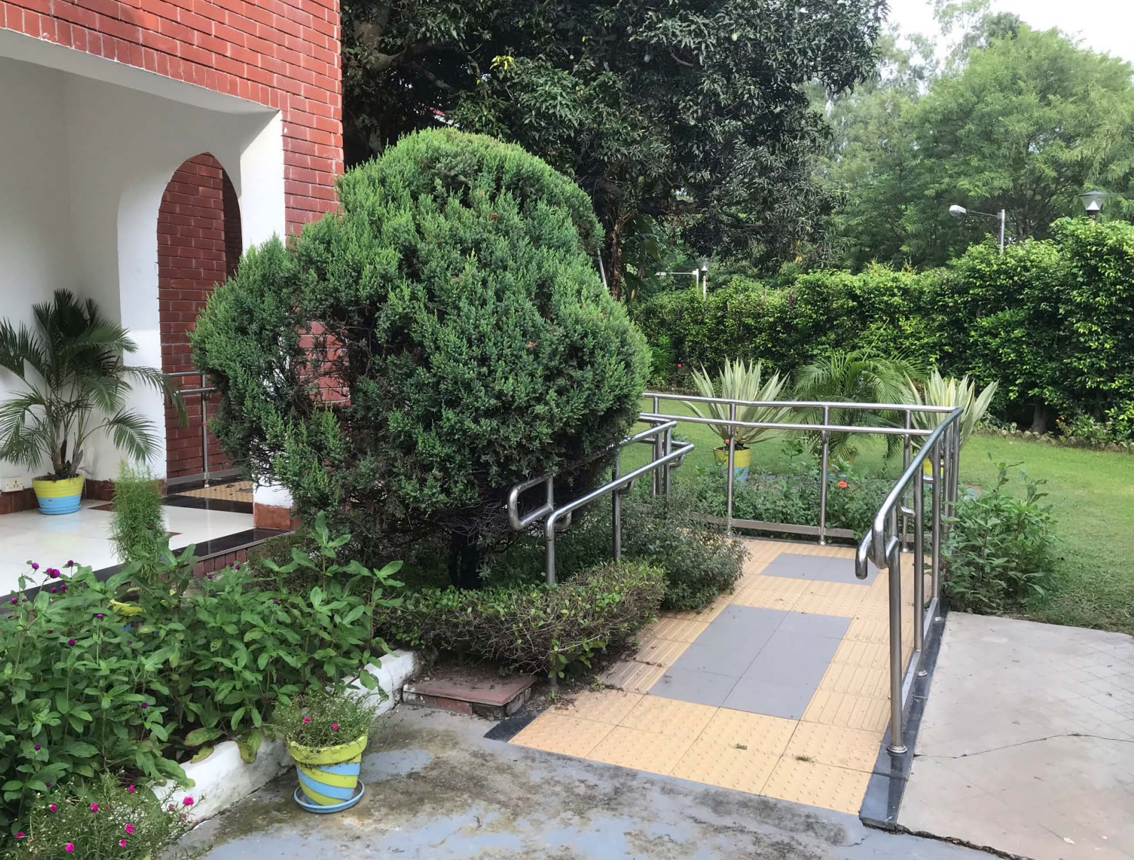
Image 7.6 Retrofitted ramp as an accessible entrance of a guest house Photo Credits: Dr. Gaurav Raheja
