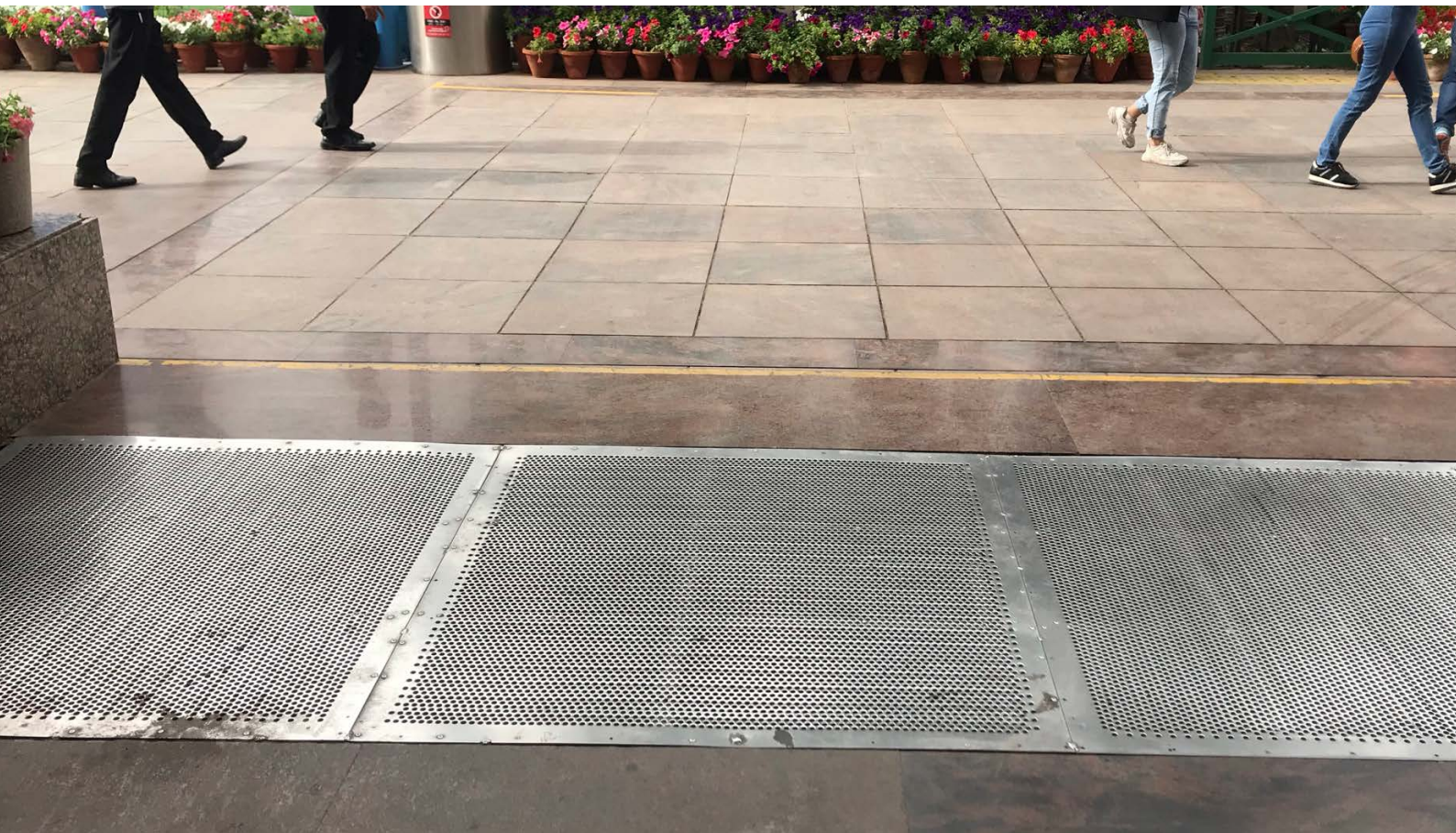
Image 3.12 Accessible grating details ( Perforated grating type) Photo Credits: Dr. Gaurav Raheja
