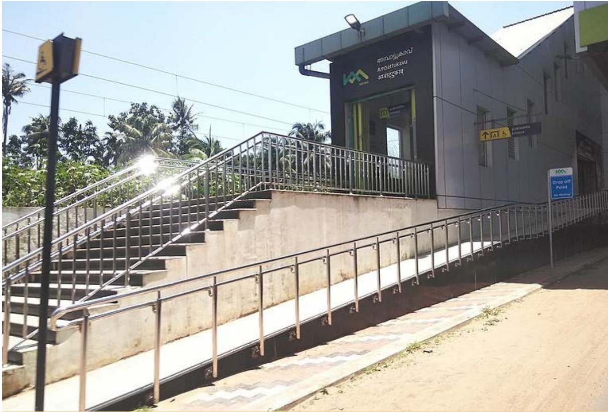
Image 6.23 Accessible metro station entrances: Kochi Metro Station Source https://en.wikipedia.org/wiki/Ambattukavu_metro_station
