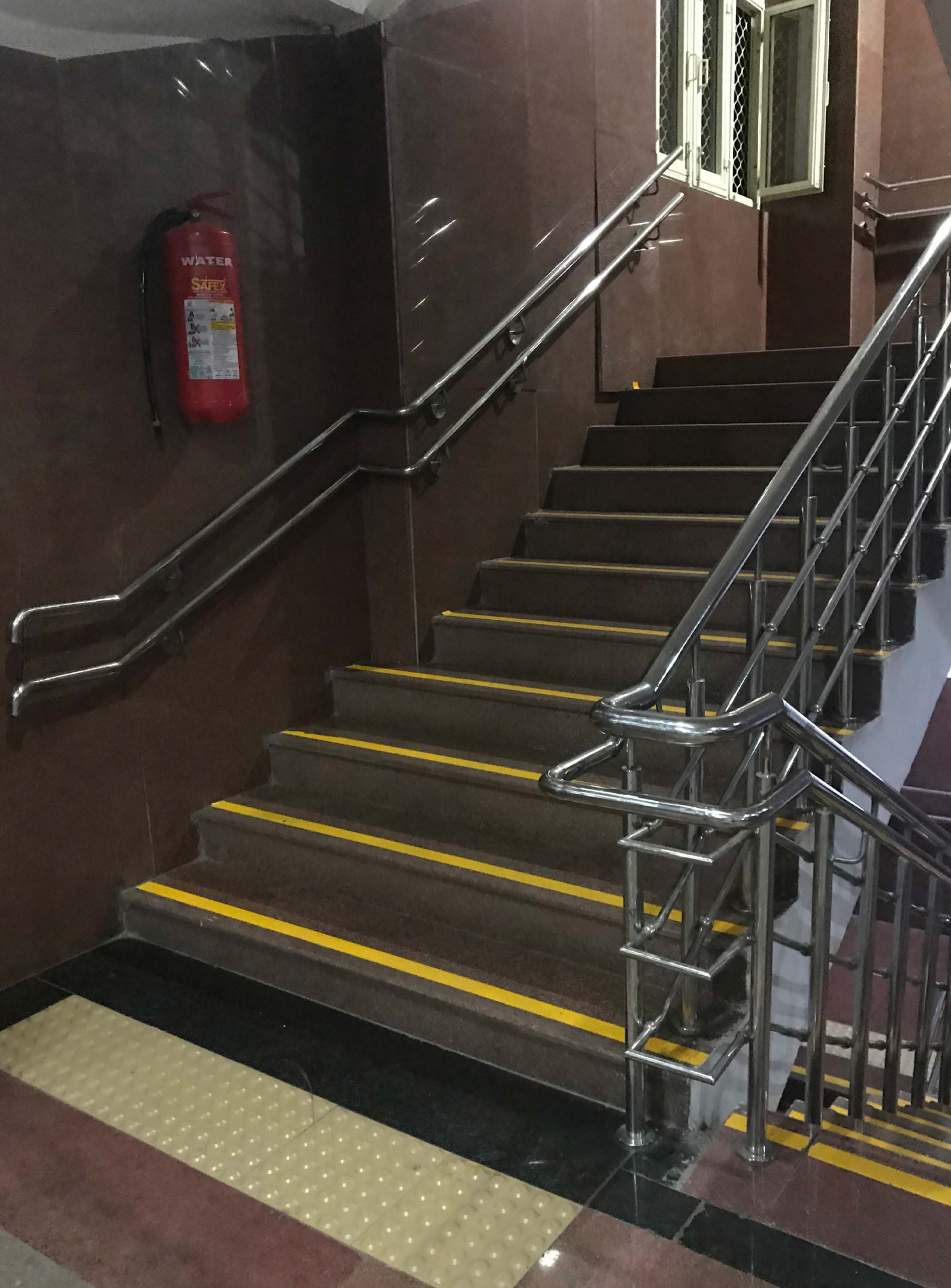
Image 4.6 Staircase with color contrast and tactile tiles Photo Credits: Dr. Gaurav Raheja
