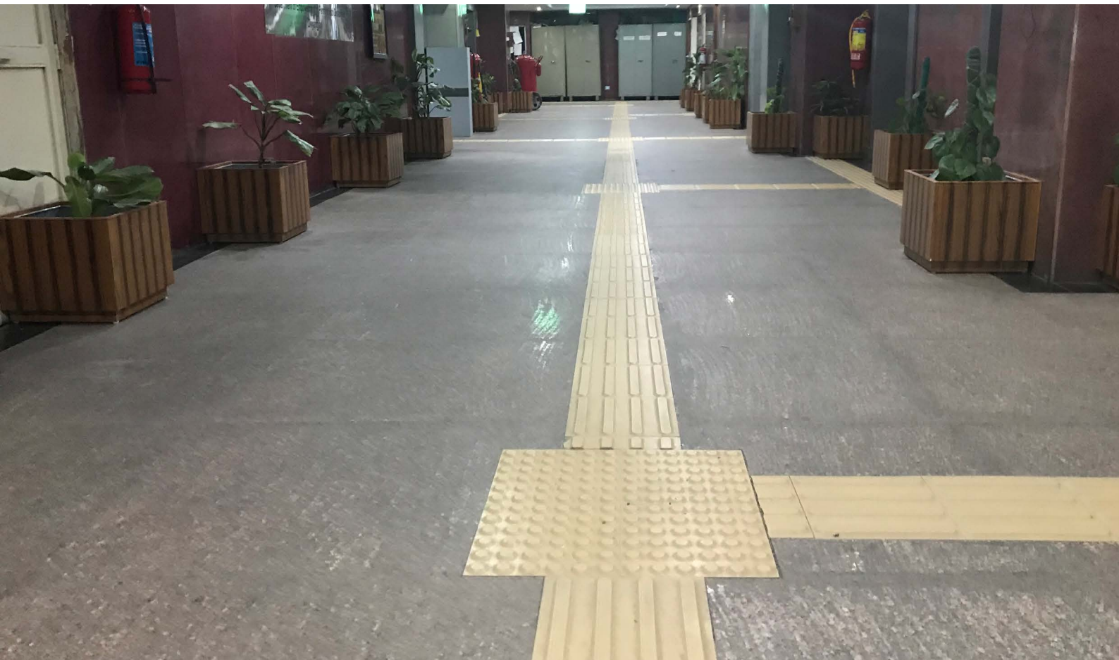
Image 4.5 Internal corridor with tactile tiles
