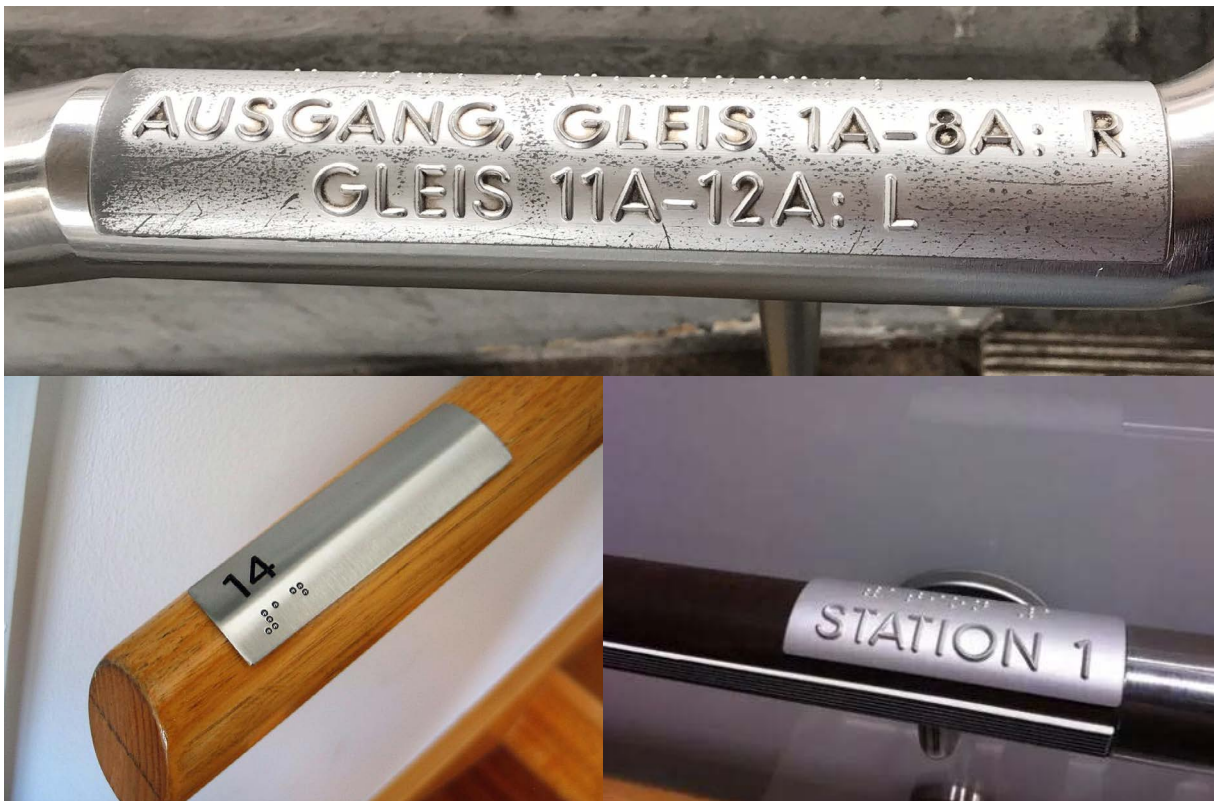
Image 5.12 Braille sign on handrail bars
