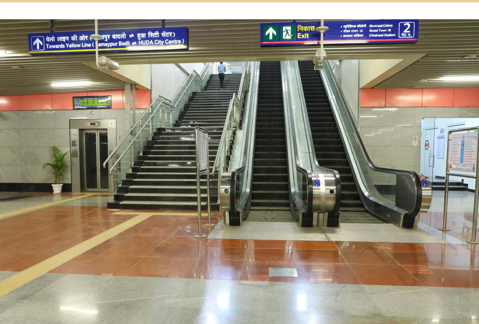
Image 6.21 Inclusive vertical circulation in train station enabled with Lift, staircase and escalator Photo Credits: DMRC
