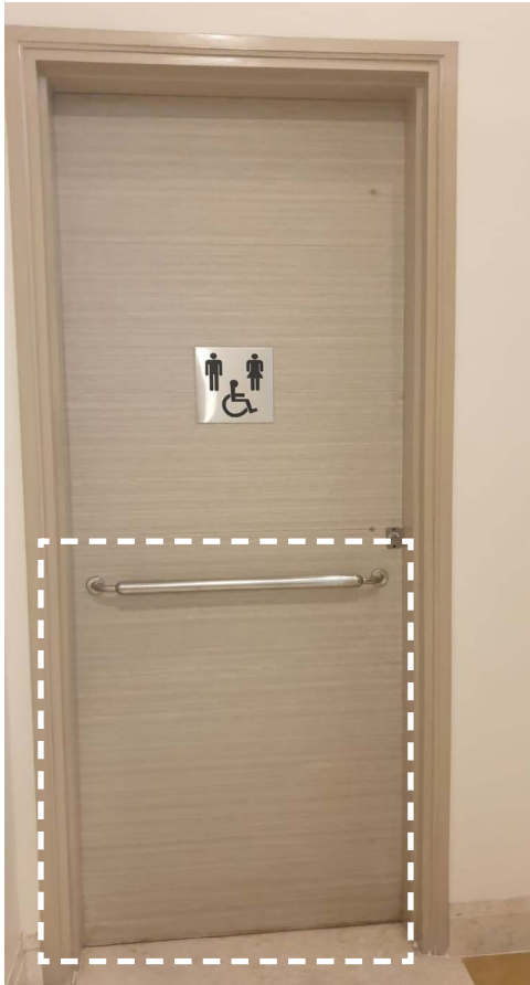
Image 2.13 Absence of kick plate and lever handle
