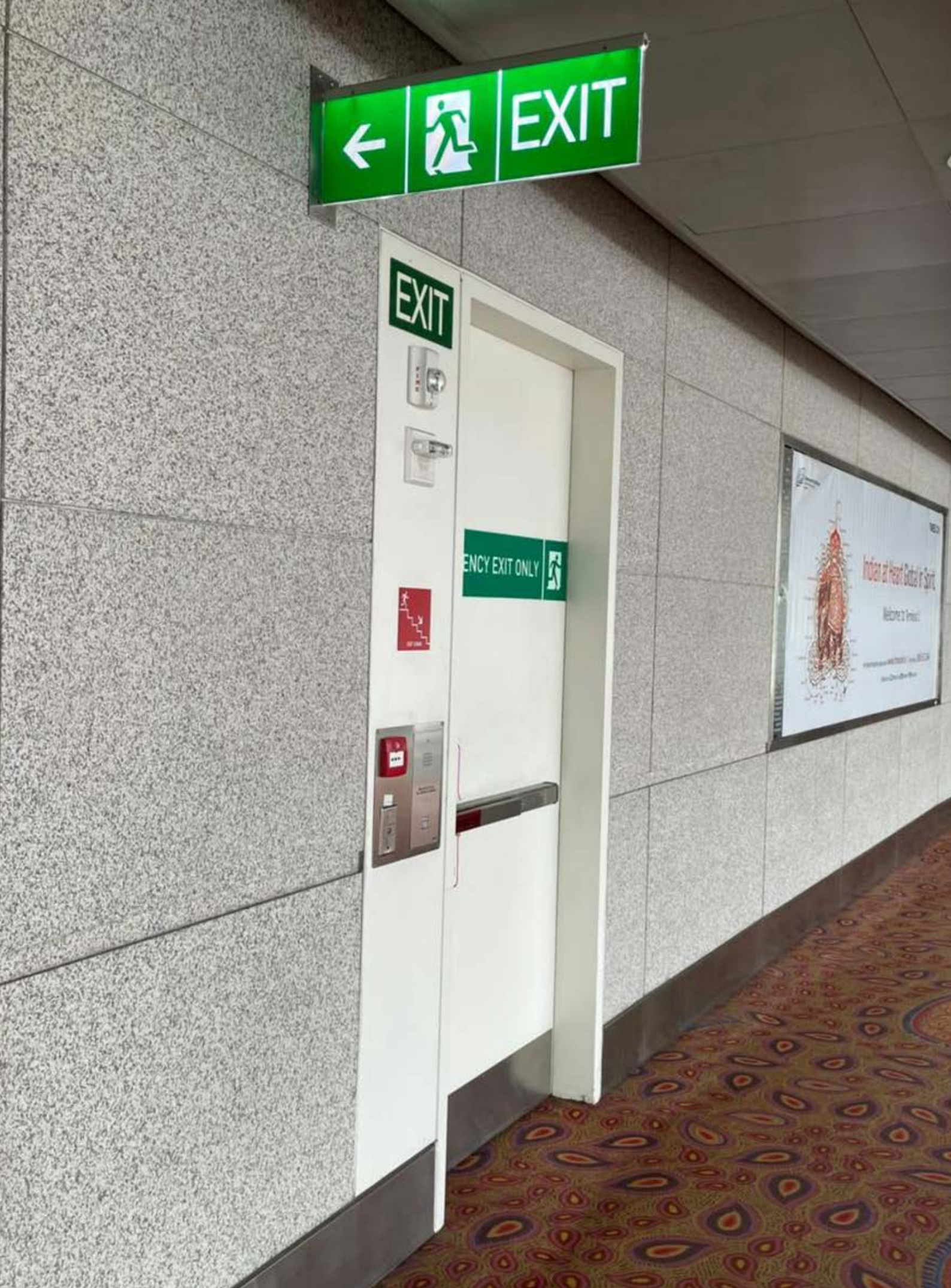
Image 7.1 Emergency exit door Photo Credits: Dr. Gaurav Raheja
