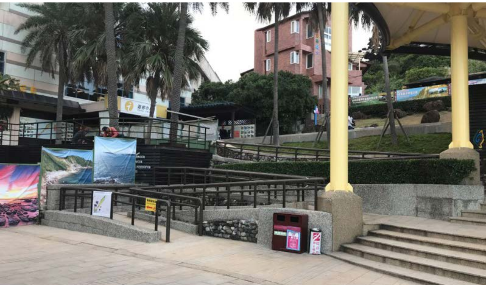
Image 3.10 Access Ramps with steps Photo Credits: Dr. Gaurav Raheja
