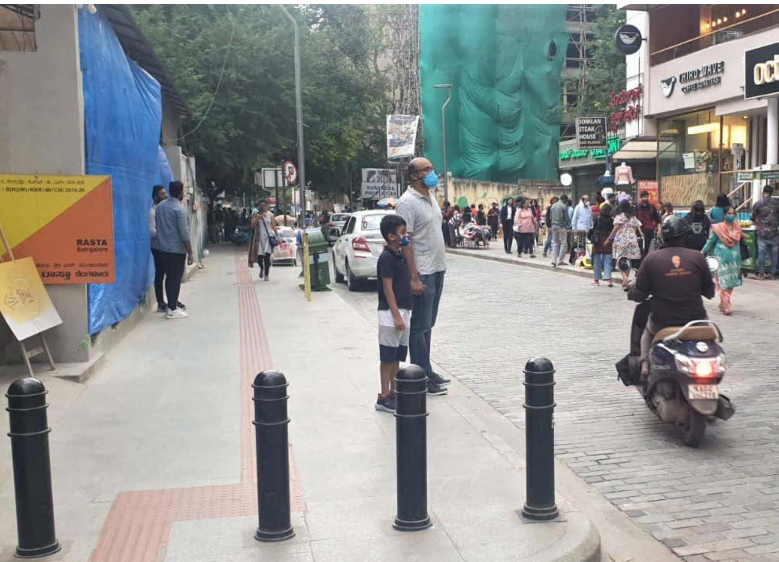
Image 3.28 Typical bollard placement for accessible sidewalk with tactile pavers: Church Street Photo Credits: Shreya Shetty
