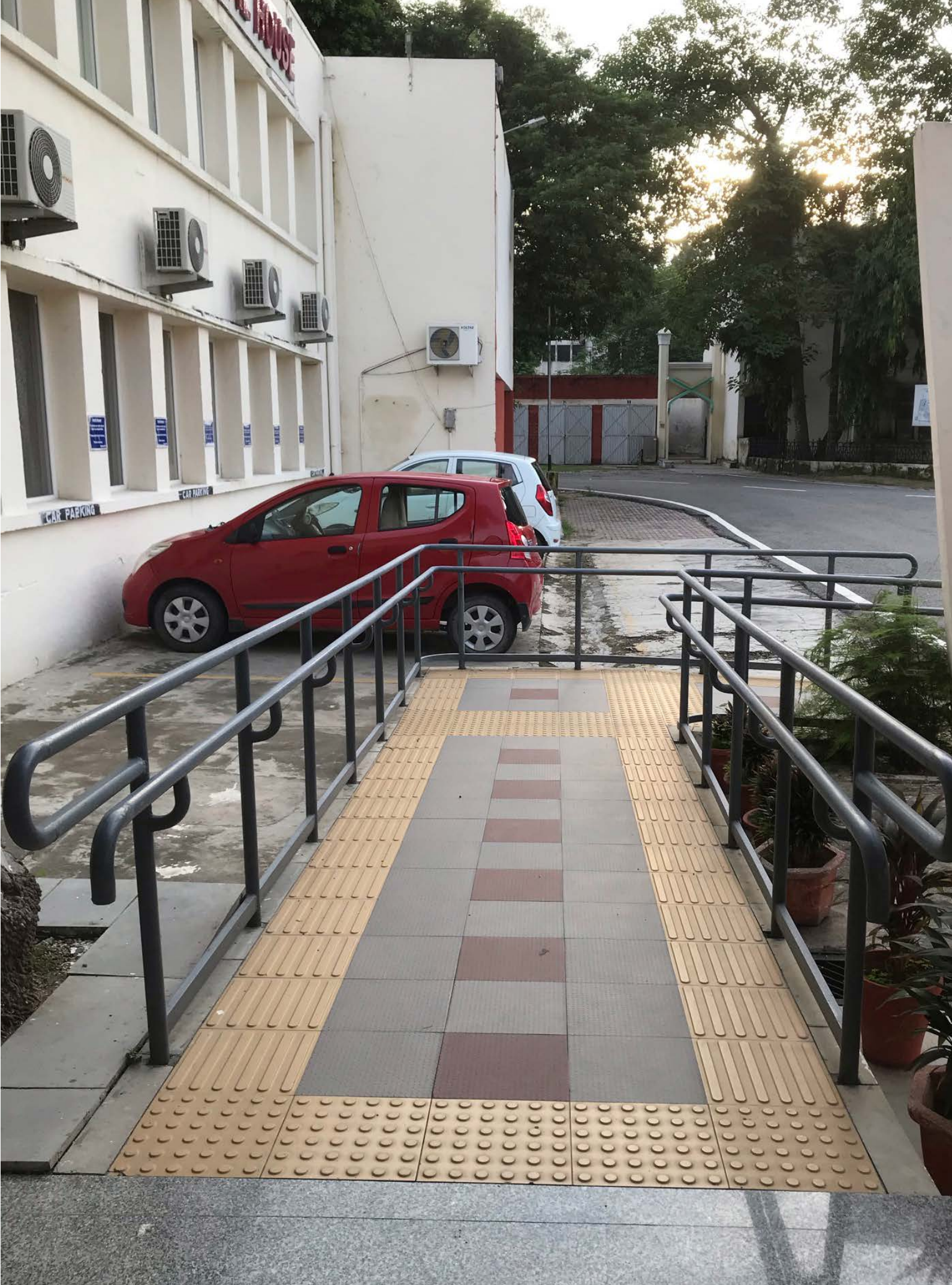
Image 3.20 Accessible ramps at building entrance Photo Credits: Dr. Gaurav Raheja
