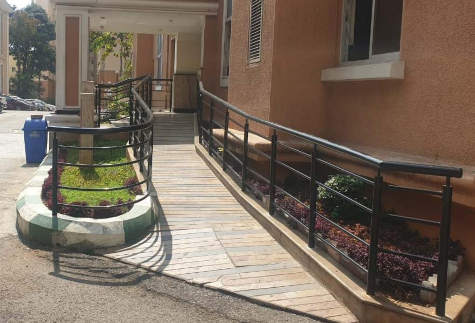
Image 6.2 Accessible ramp at the entrance of an apartment building Photo Credits: Shreya Shetty
