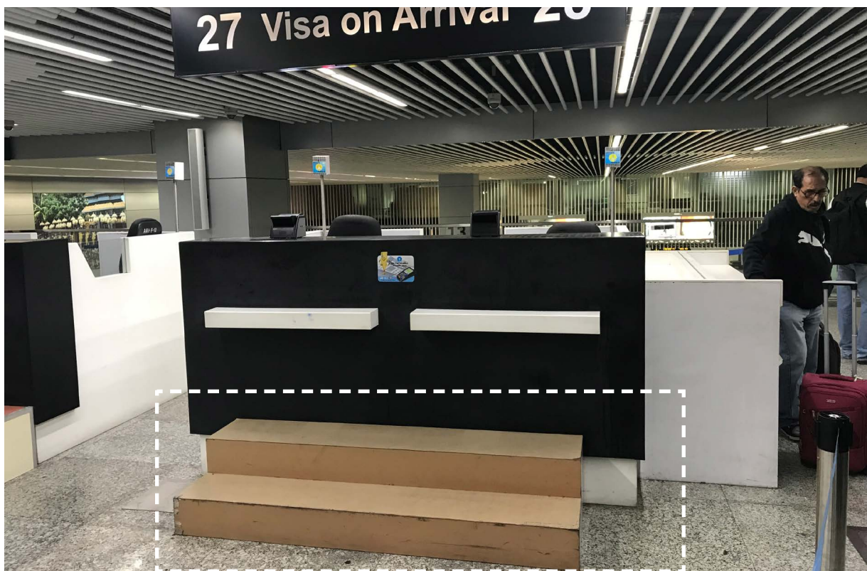
Image 2.25 Inaccessible counter heights
