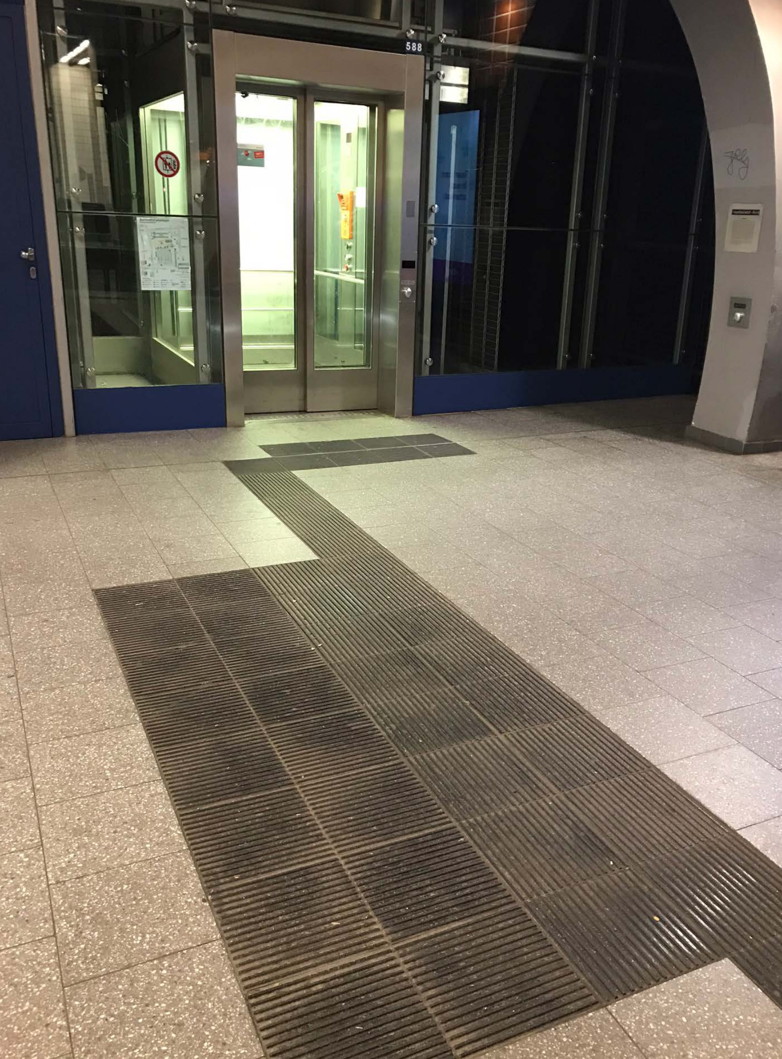
Image 4.9 Tactile pavers layout towards the lifts access Photo Credits: Dr. Gaurav Raheja
