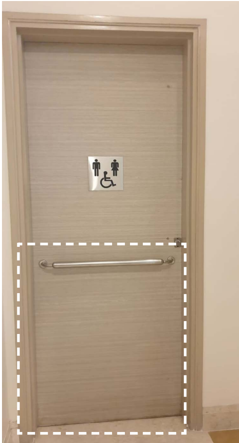
Image 2.13 Absence of kick plate and lever handle
