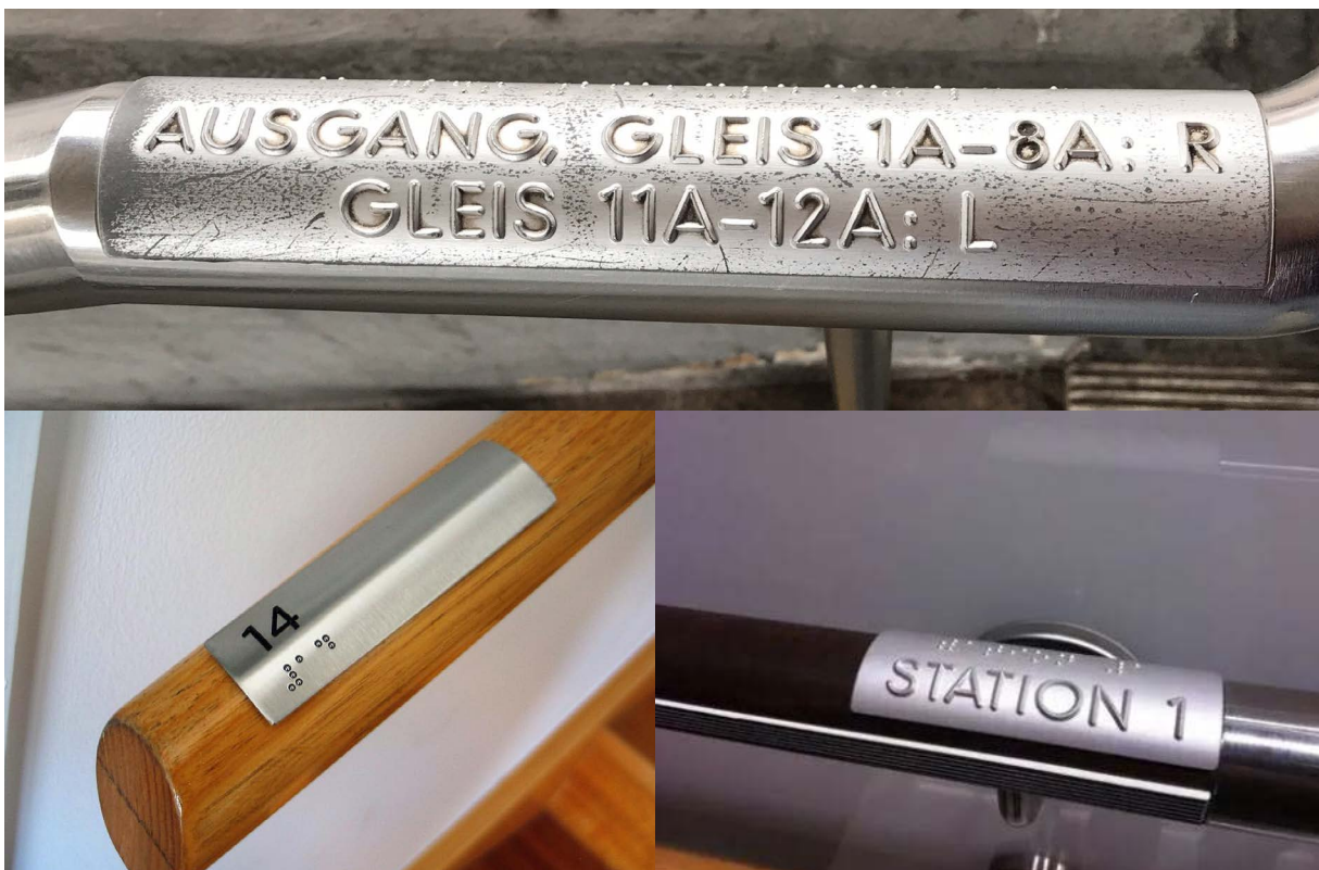
Image 5.12 Braille sign on handrail bars
