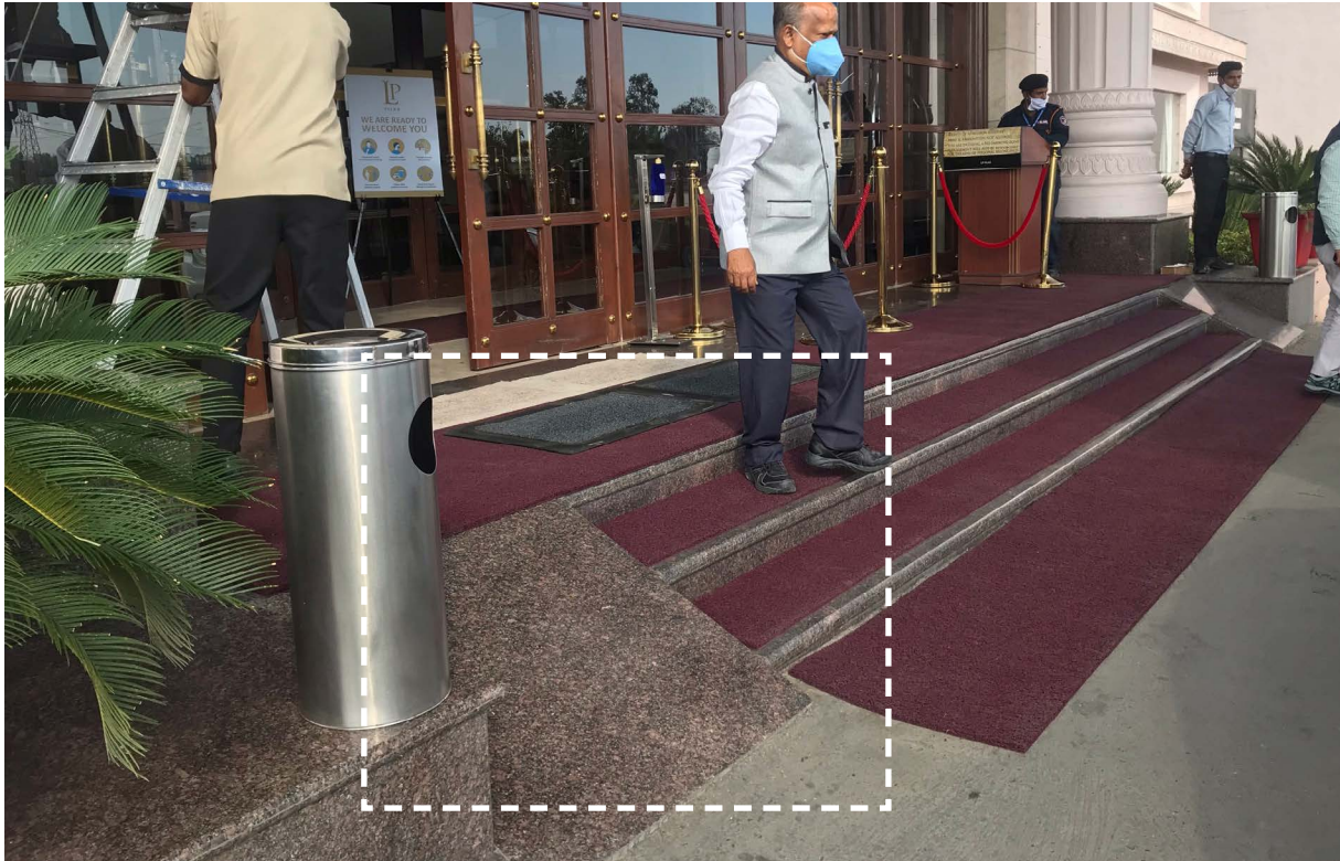
Image 2.7 Improper ramp gradient and slippery floor finish
