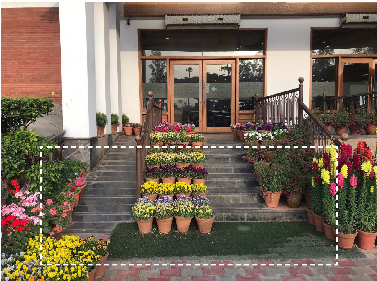
Image 2.12 Planters as barrier and inadequate ramp slope
