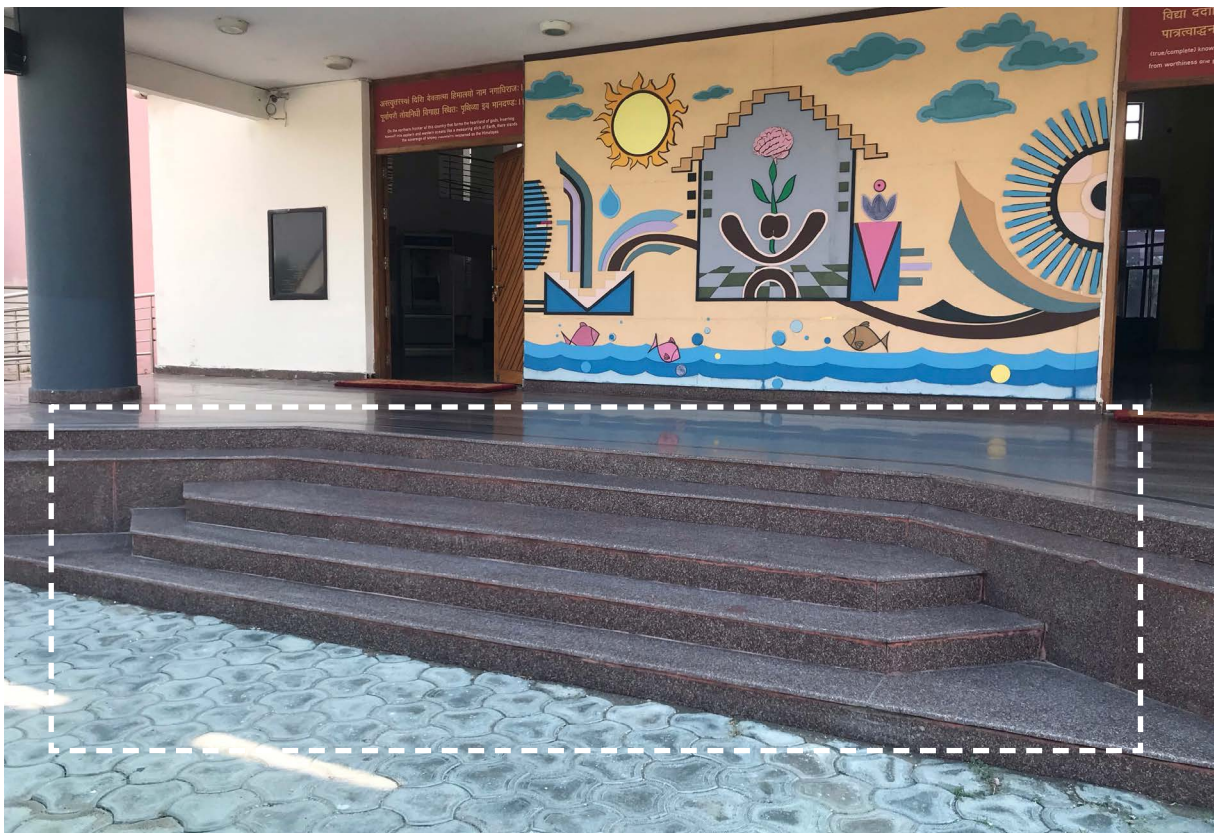
Image 2.3 Absence of adequate visual contrast in steps
