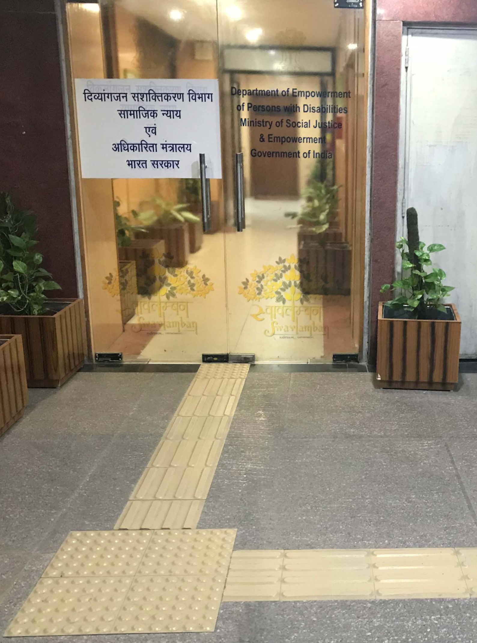
Image 3.19 TGSi pathway in horizontal circulation Photo Credits: Dr. Gaurav Raheja
