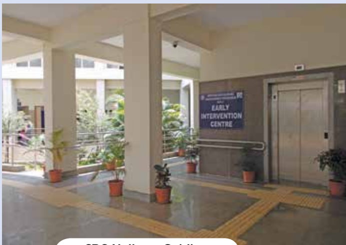
CRC Nellore: Guiding Tactile and Handrails to Accessible Lift
