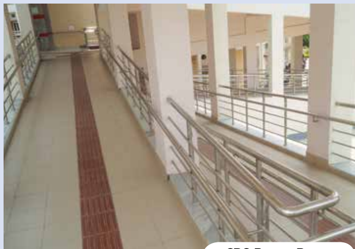
CRC Patna: Ramp with Guiding Tactile and Handrails
