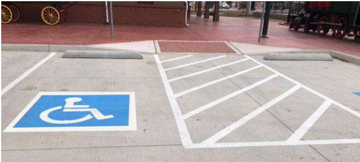
Image 1: Example of parking symbol on floor, transfer bay marking and kerb ramp
