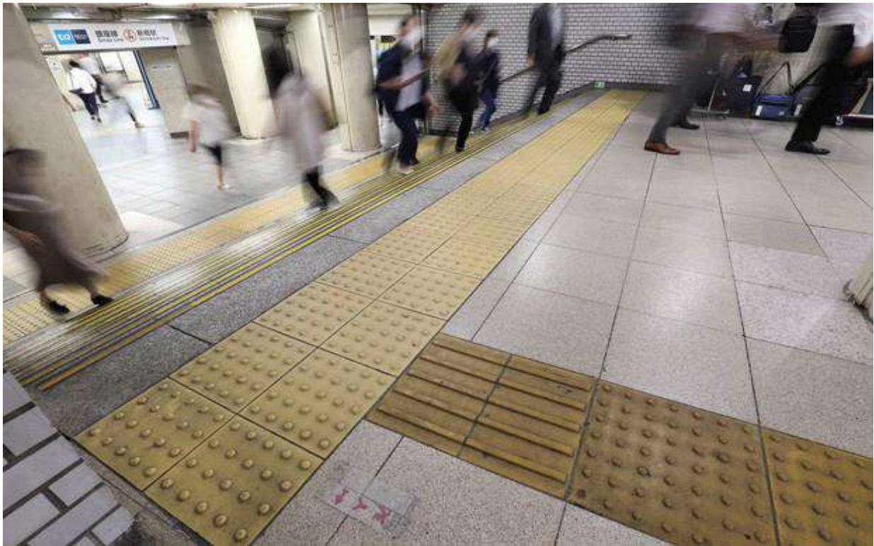
Image 9: Example of tactile flooring provided at the beginning of the staircase
