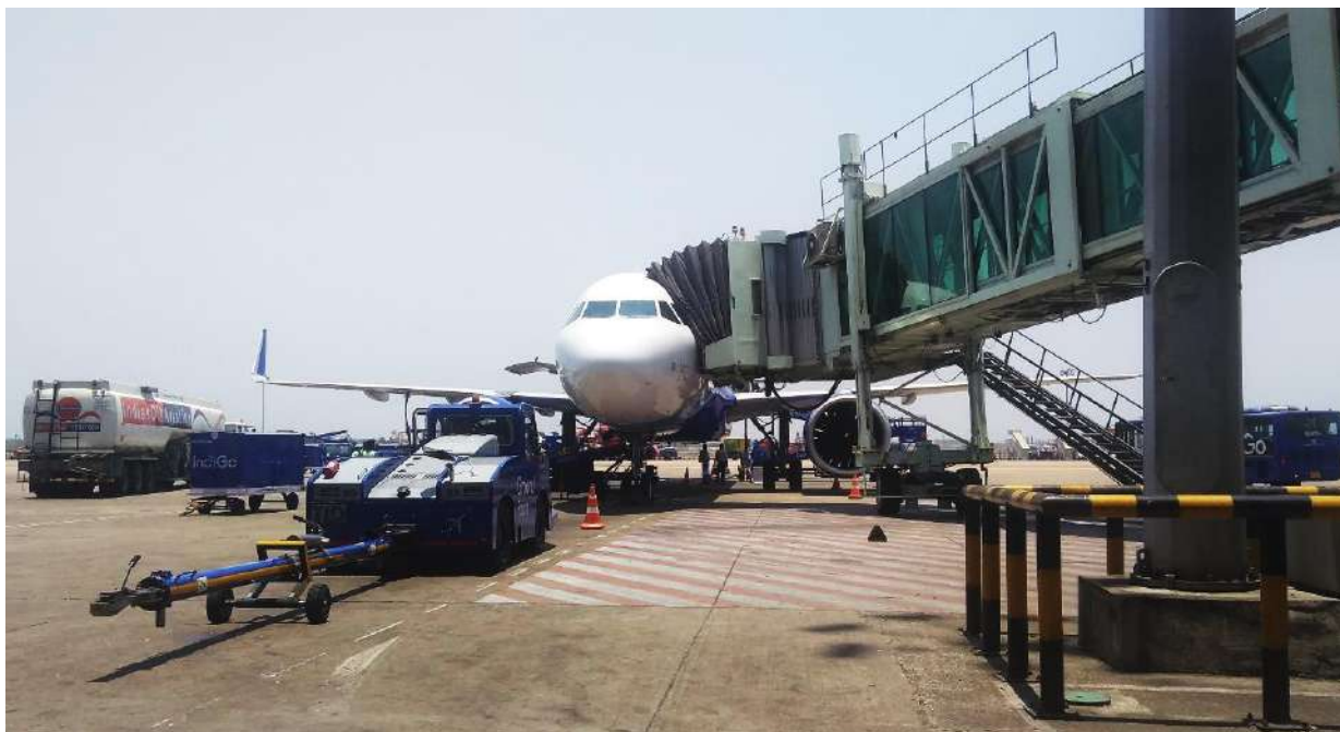
Image 21: Example of aerobridge at Chennai Airport
