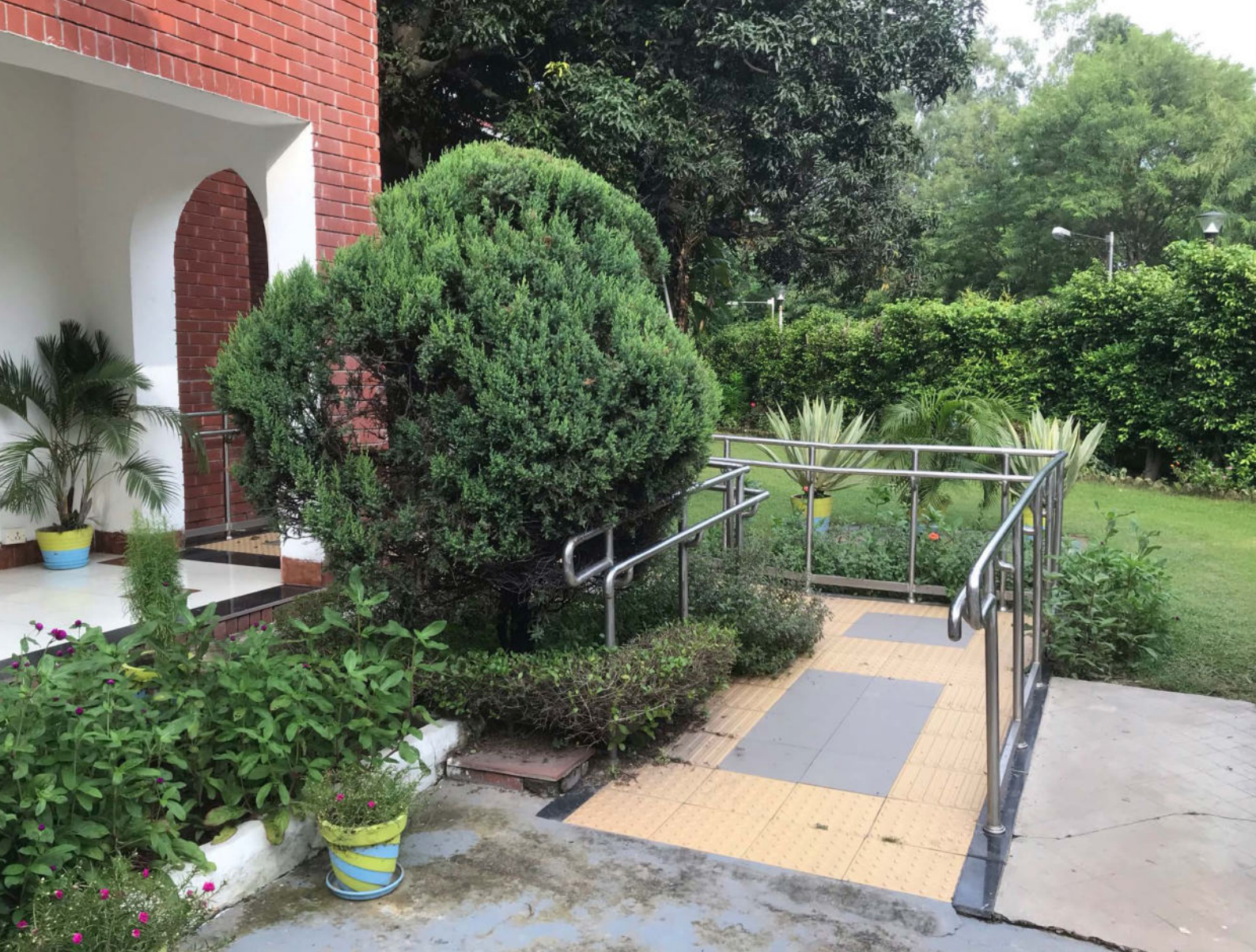
Image 7.6 Retrofitted ramp as an accessible entrance of a guest house Photo Credits: Dr. Gaurav Raheja
