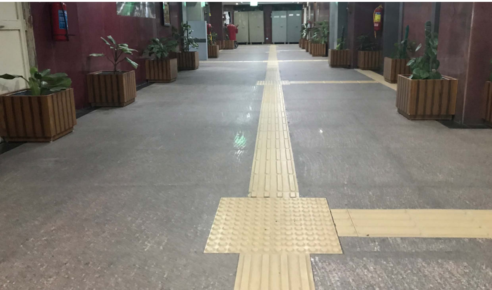
Image 4.5 Internal corridor with tactile tiles Photo Credits: Dr. Gaurav Raheja
