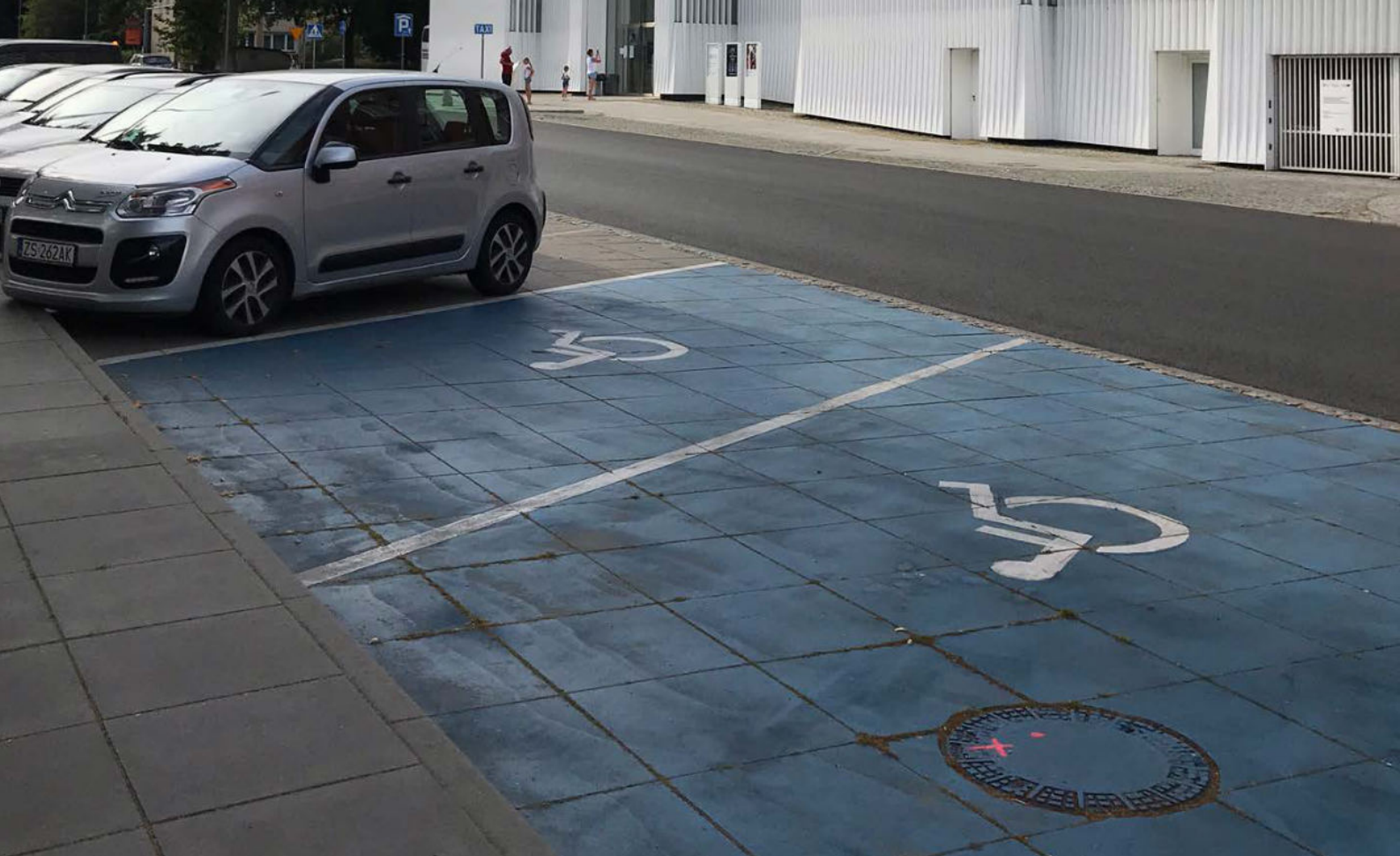
Image 3.4 Accessible reserved parking bays Photo Credits: Dr. Gaurav Raheja
