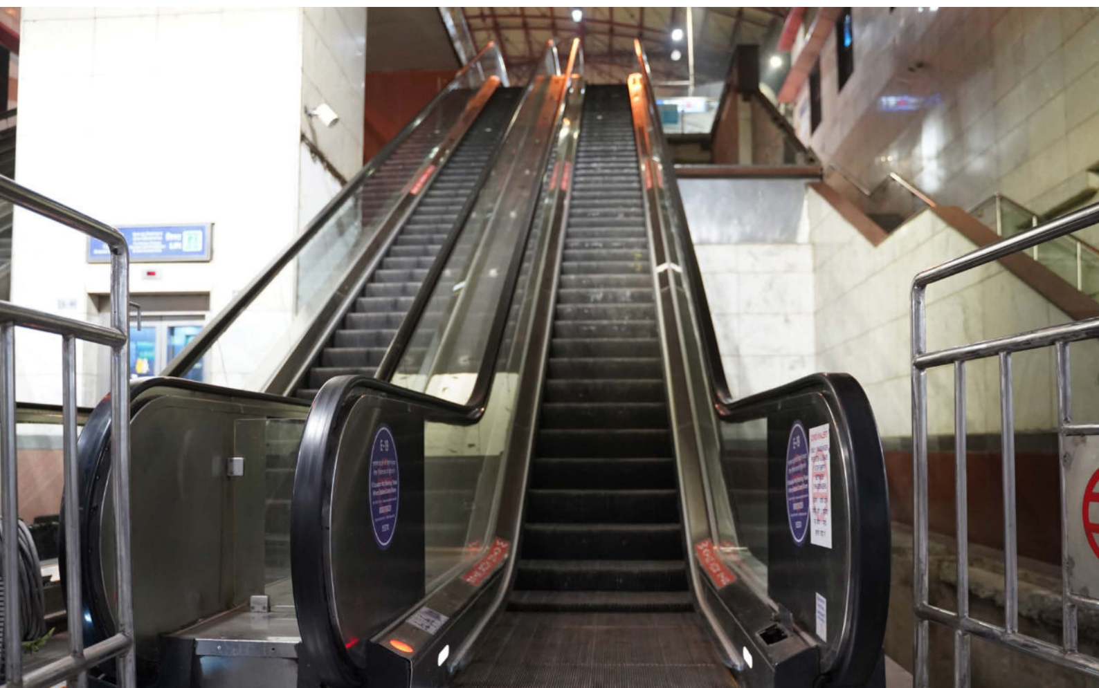
Image 3.22 Handrails as support in accessible staircase and escalators Photo Credits: DMRC, New Delhi
