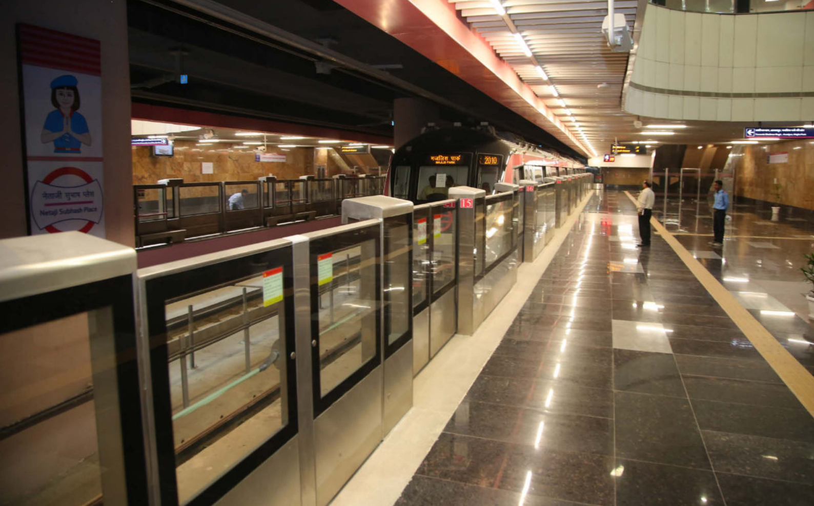
Image 6.20 Leveled approach on accessible train platform Photo Credits: DMRC
