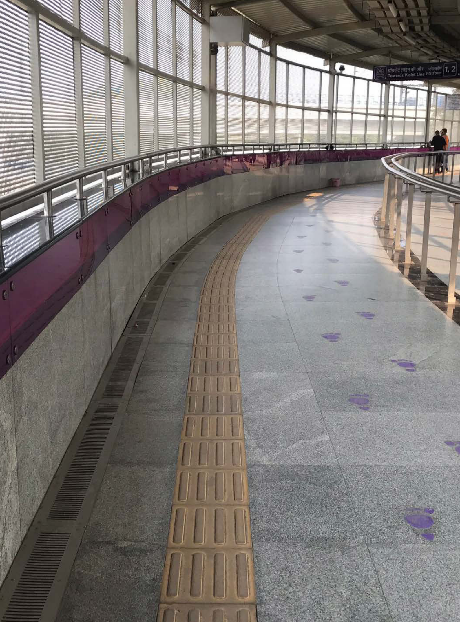
Image 3.21 Accessible horizontal circulation with handrail
