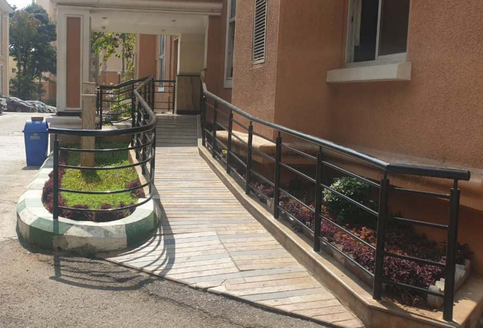
Image 6.2 Accessible ramp at the entrance of an apartment building Photo Credits: Shreya Shetty
