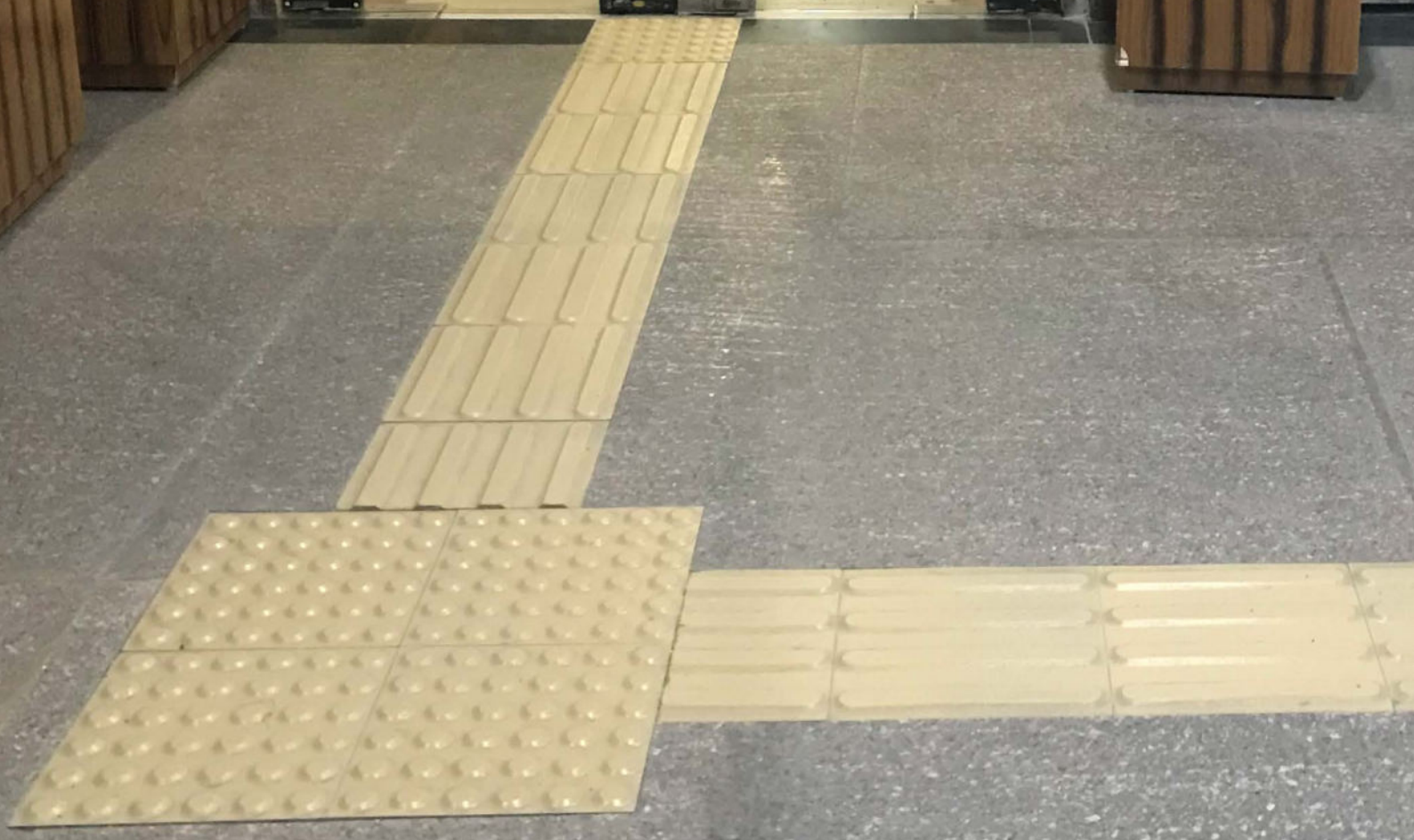
Image 3.19 TGSi pathway in horizontal circulation Photo Credits: Dr. Gaurav Raheja
