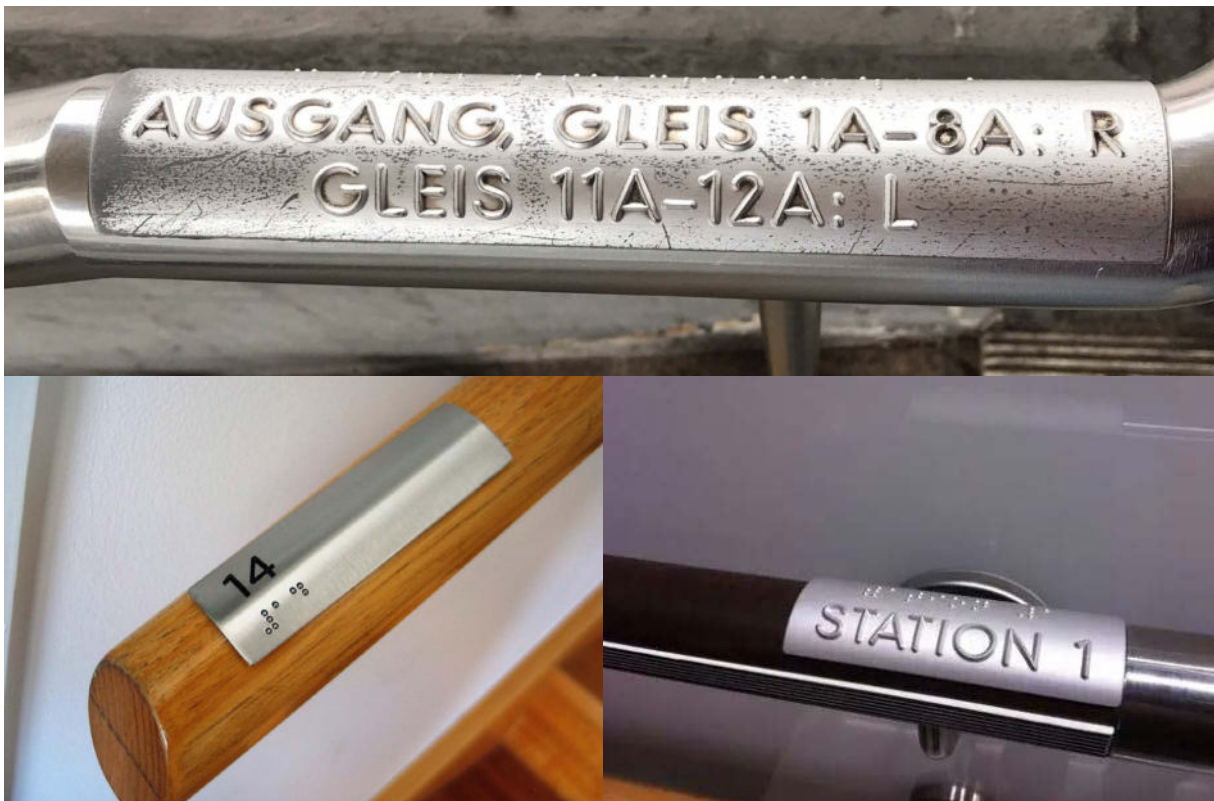
Image 5.12 Braille sign on handrail bars
