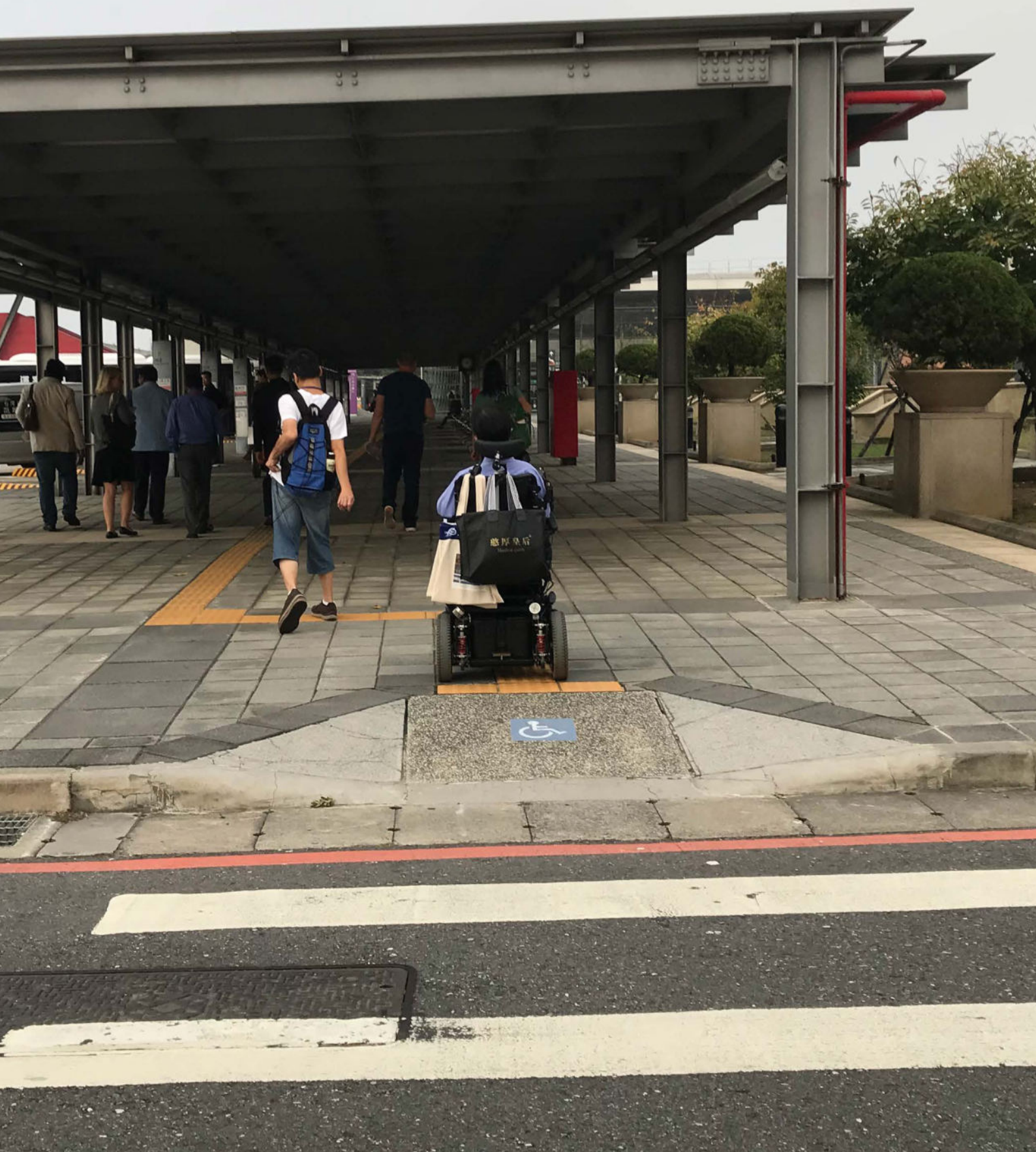
Image 3.13 Accessible flared kerb ramp at pedestrian crossing Photo Credits: Dr. Gaurav Raheja
