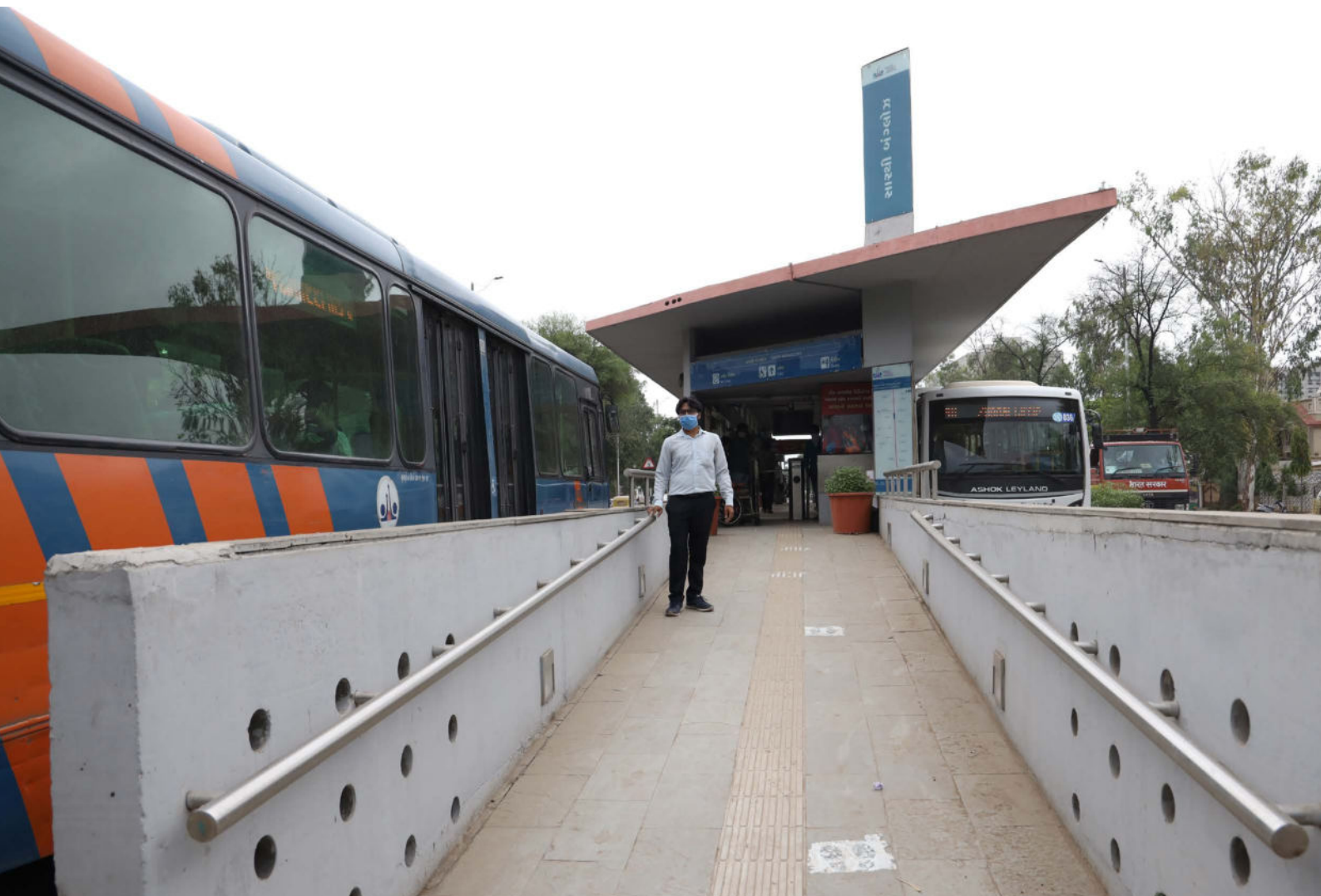
Image 6.11 Accessible approach for bus shelter Photo Credits: CPWD
