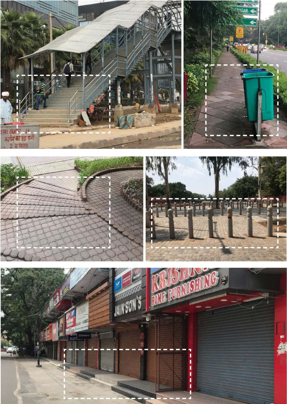
Image 2.26 Typical Barrier in built environment
