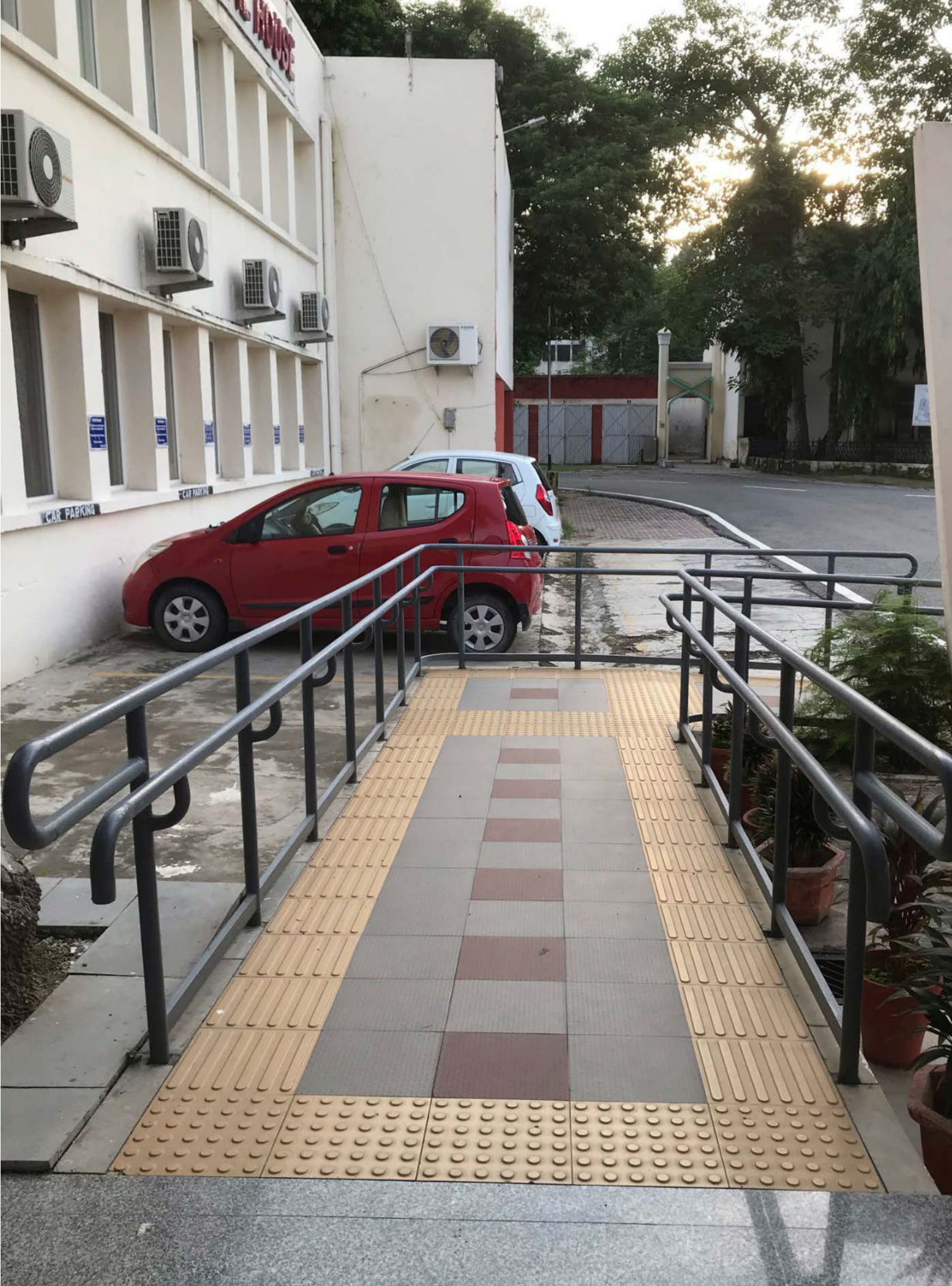
Image 3.20 Accessible ramps at building entrance
