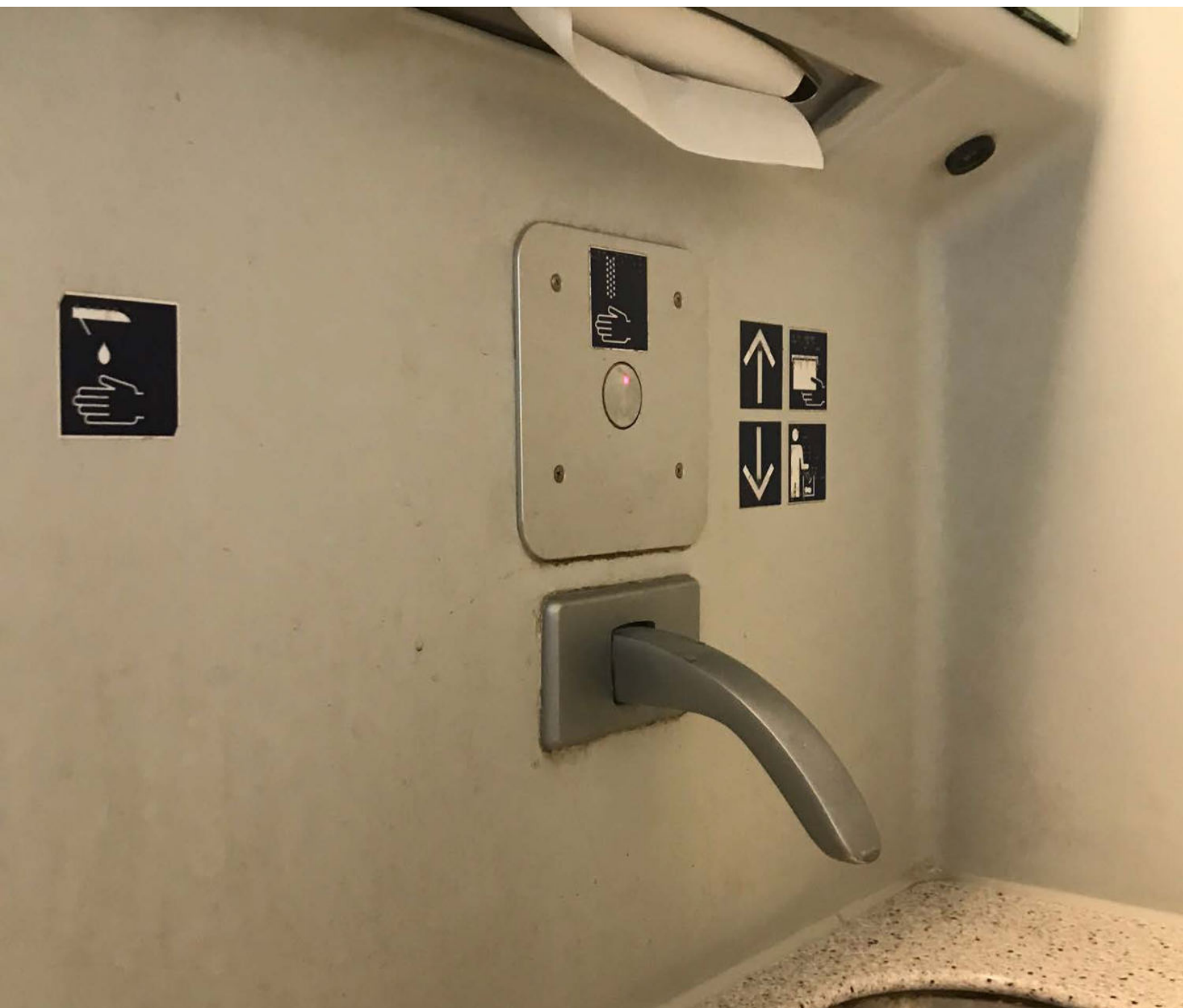
Image 4.22 Accessible sensor based faucet Photo Credits: Dr. Gaurav Raheja
