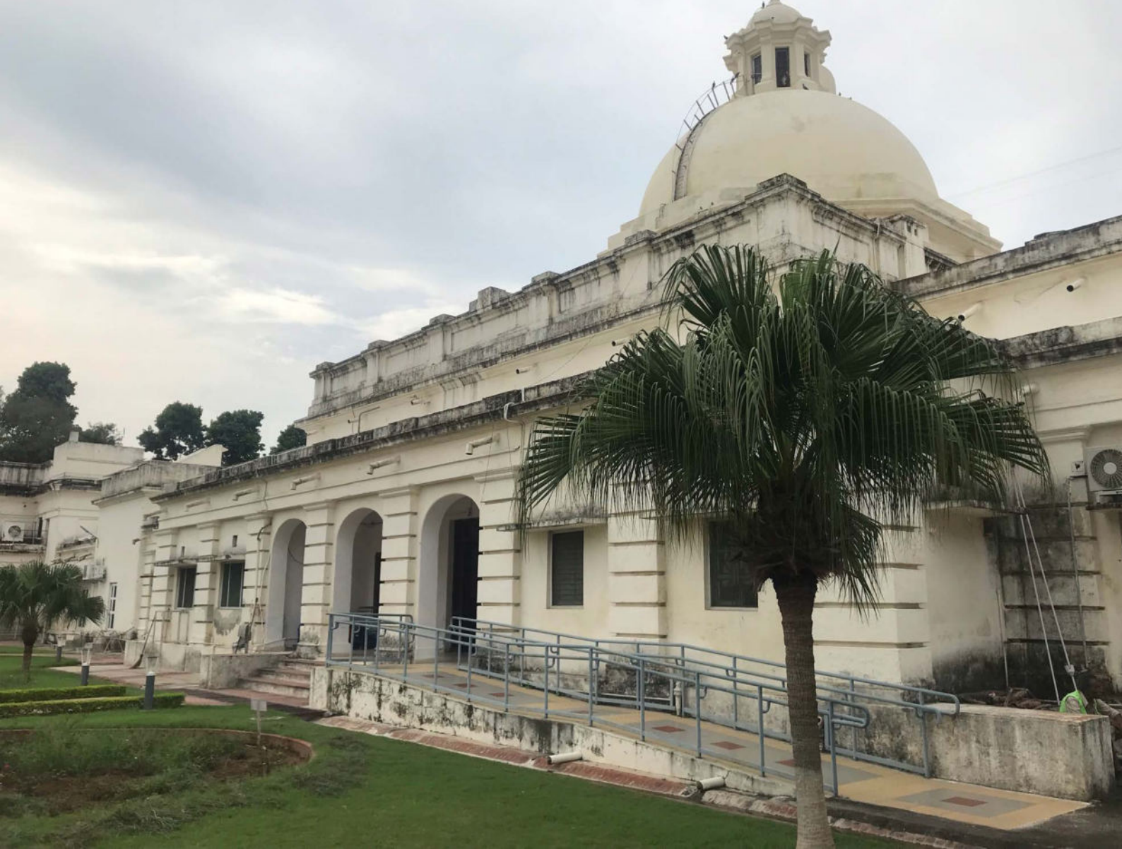
Image 7.7 Retrofitted accessible entrance through ramps in a heritage building Photo Credits: Dr. Gaurav Raheja
