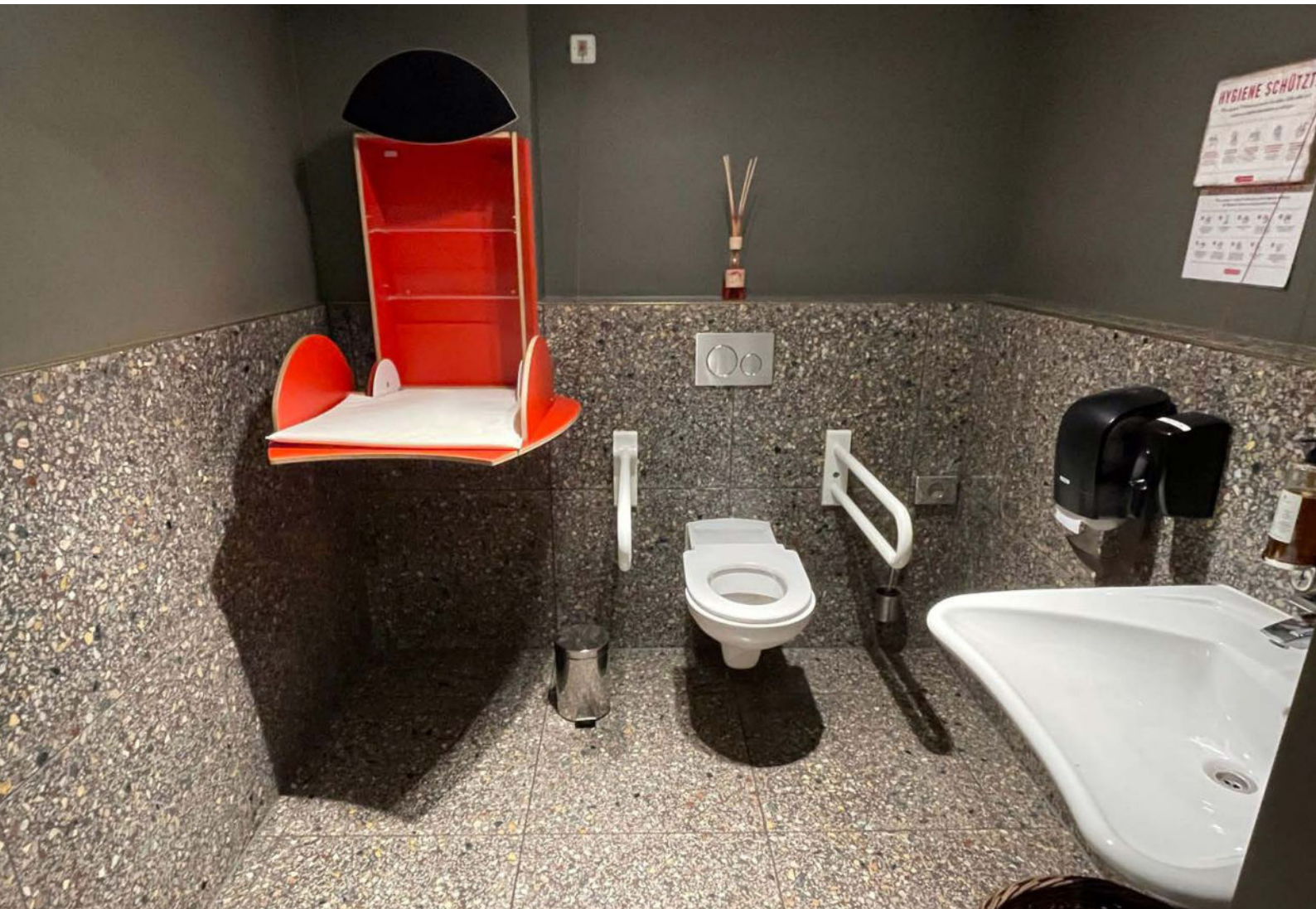
Image 4.28 Accessible Washroom with diaper changing station Photo Credits: Dr. Gaurav Raheja
