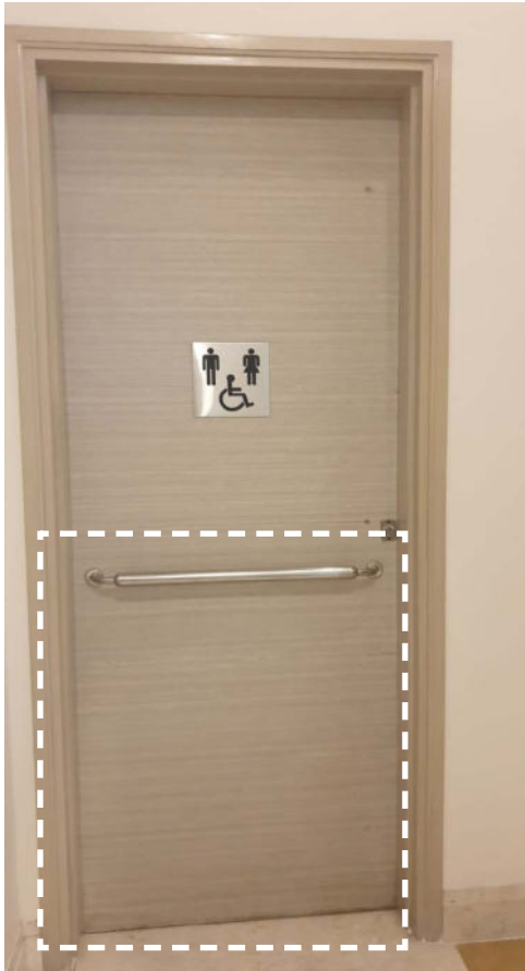
Image 2.13 Absence of kick plate and lever handle
