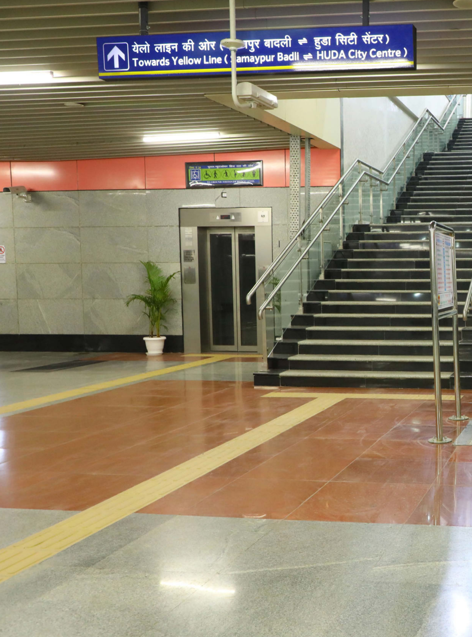
Image 3.17 Accessible transportation environment with Tactile Pavers with good visual contrast Photo Credits: DMRC, New Delhi
