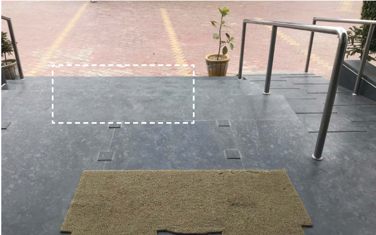
Image 2.18 Poor visual contrast in entrance steps
