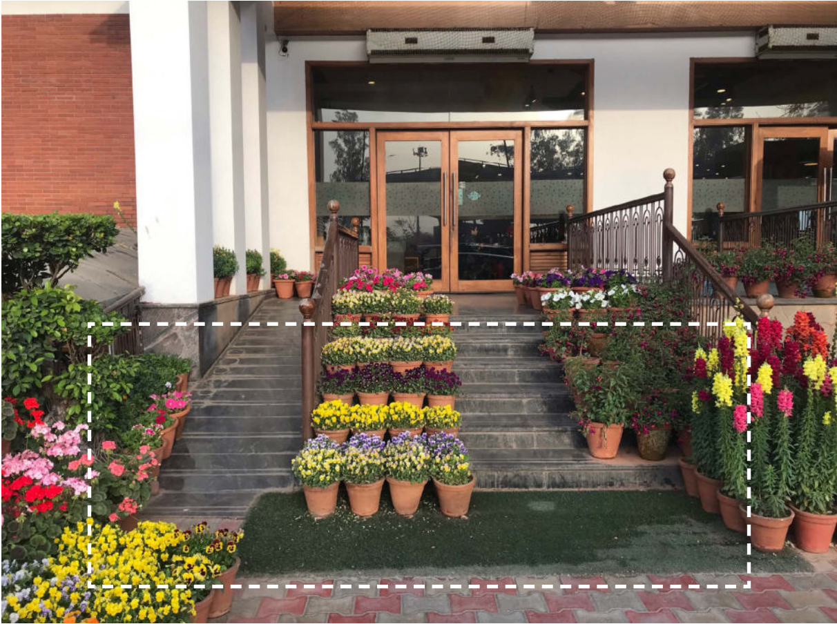
Image 2.12 Planters as barrier and inadequate ramp slope
