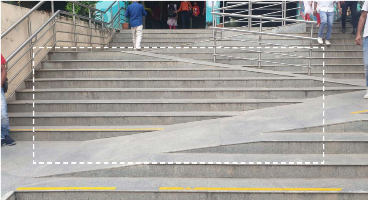
Image 2.11 Inadequate colour contrast
