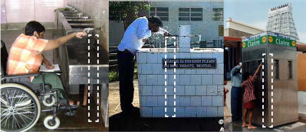
Image 2.16 Inaccessible heights for wheelchair users and children
