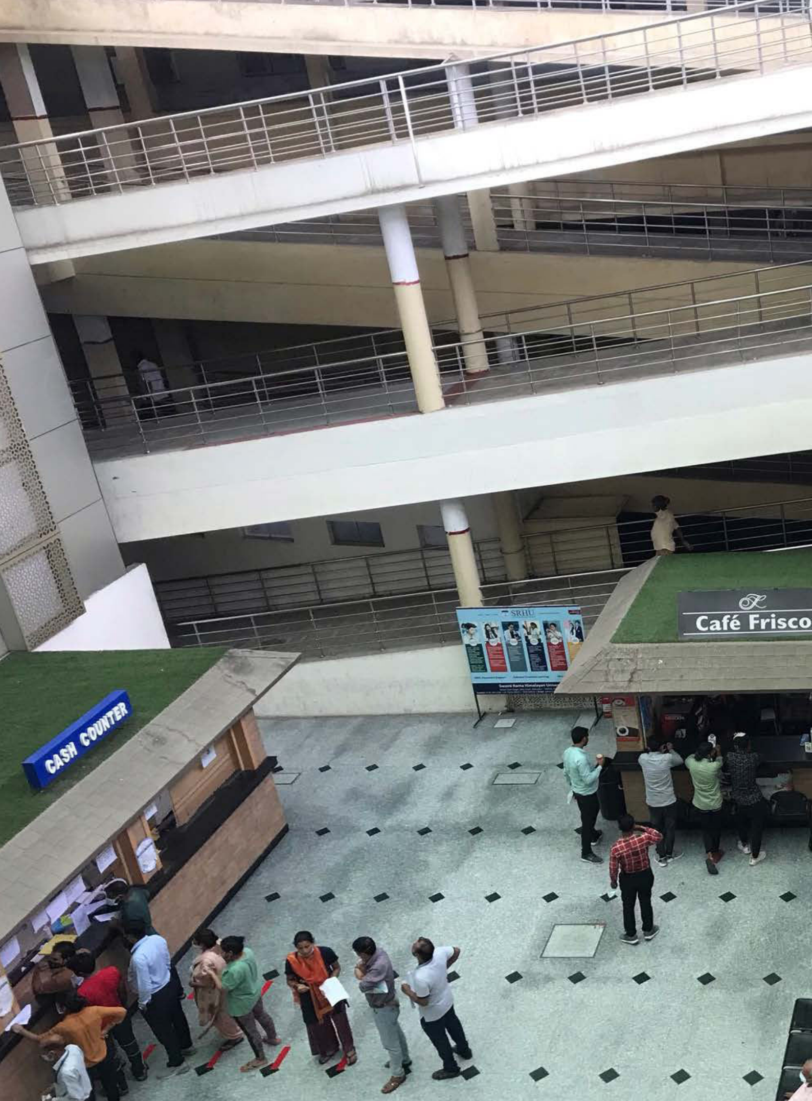
Image 6.37 Accessible internal ramp in the hospital Photo Credits: Dr. Gaurav Raheja
