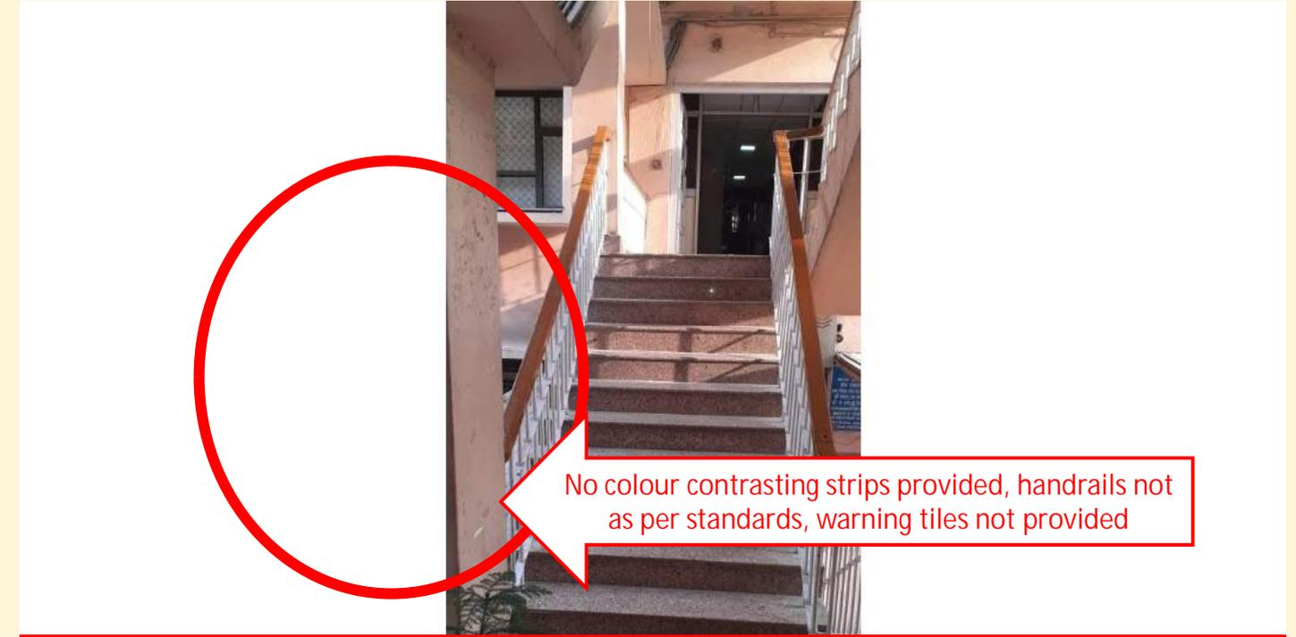
No colour contrasting strips provided, handrails not as per standards, warning tiles not provided
