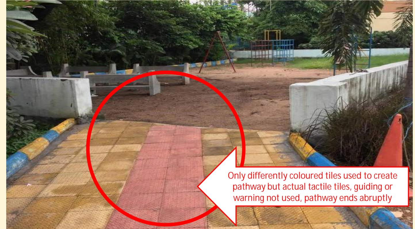
Only differently coloured tiles used to create pathway but actual tactile tiles, guiding or warning not used, pathway ends abruptly
